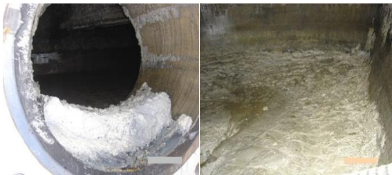
Fig. 1 Examples of clays observed in the production tanks and pipelines
