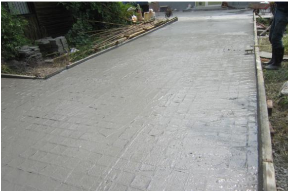
(c) The concrete pouring
