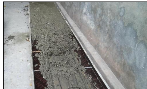
Figure 4: Concrete pouring in formwork for panel
