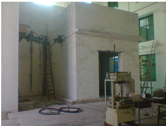
Figure 2: Repaired Specimen after non engineered conventional repair
