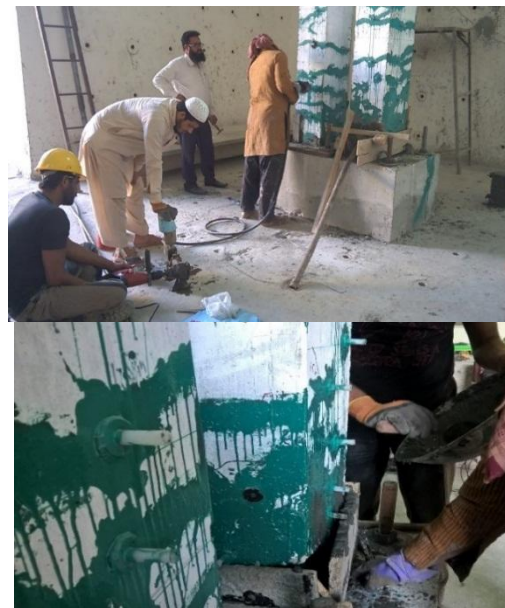
Figure 6: Epoxy Injection and Patching of Spalled Concrete
