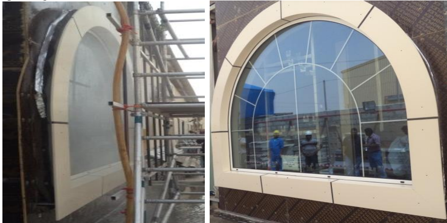
Figure 3: Window subjected to water pressure (Left), Window after the testing (Right)
