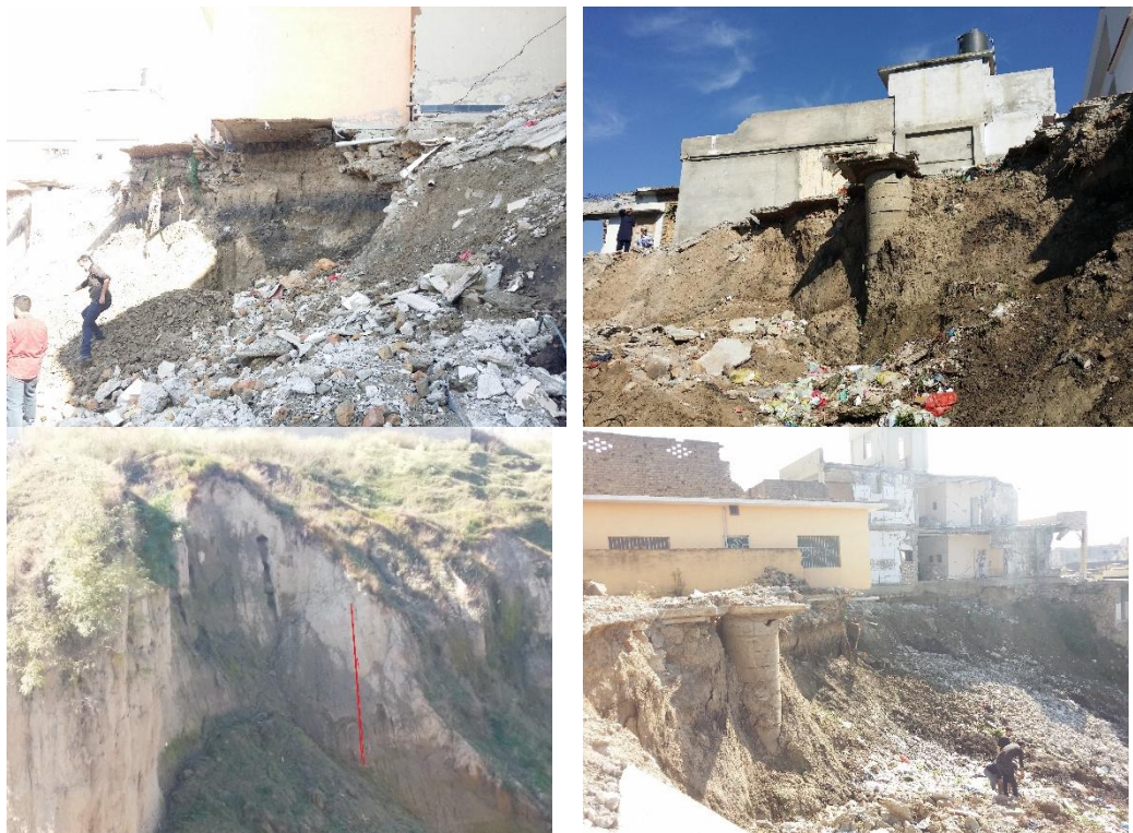
Figure 1 Landslide area of target site and residential structures effected
