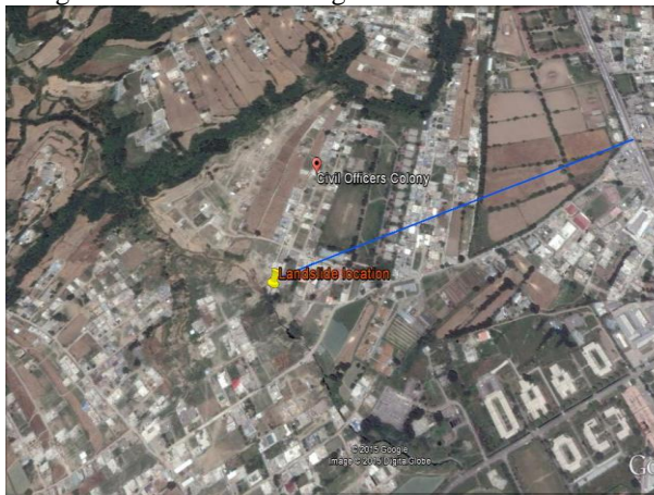
Figure 2 Location of landslide on Google Earth
