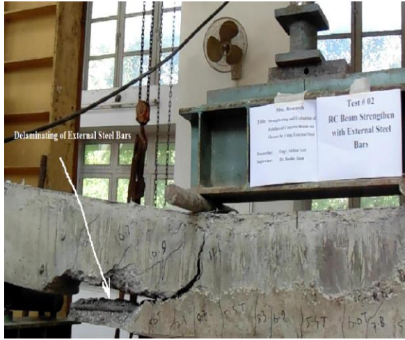
Figure: 08 Failure of Beam Strengthened with External Steel Bars
