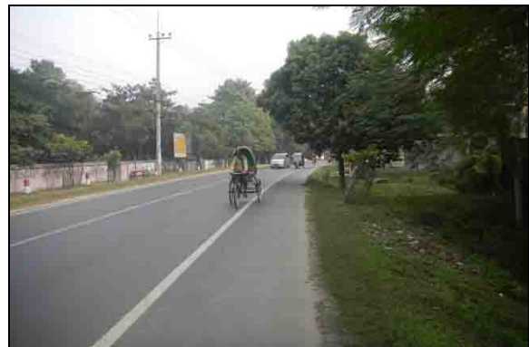
Figure 12: Inadequate horizontal clearance at the place of curve in front of Rajshahi University
