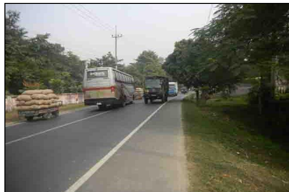
Figure 13: Serious conflict may occur due to inadequate horizontal clearance at the place of curve
