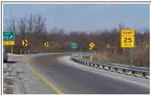
Figure 18: Adequate horizontal clearance at the place of curve
