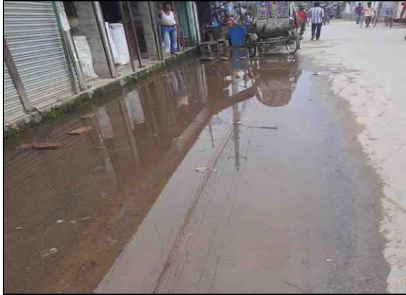
Figure 2: Water logging situation on New Market to Nagar Bhaban road due to absence of drainage system
