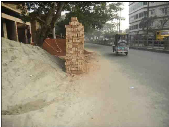
Figure 11: Shoulder is blocked by construction material both side of the road at Vodra
