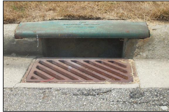
Figure 15: Road with surface drainage
